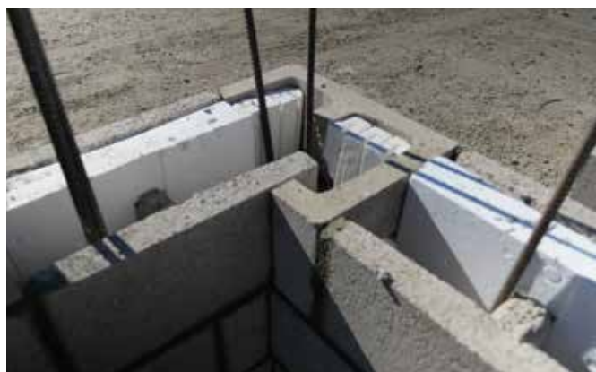
A traditional 12x8x16 CMU cut to convert it into a corner unit.
