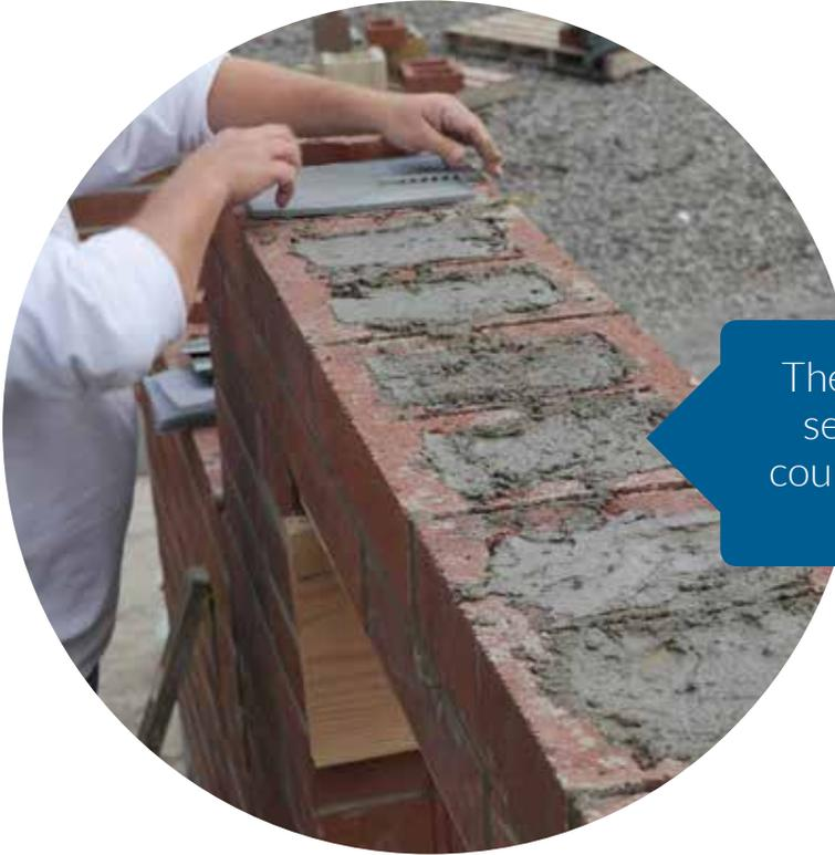
At this point, the bond beam units course is laid. After placement of the rebar in the bond beam units, the second course of Spec-Brik WCT units is laid, and the entire assembly is then grouted.
