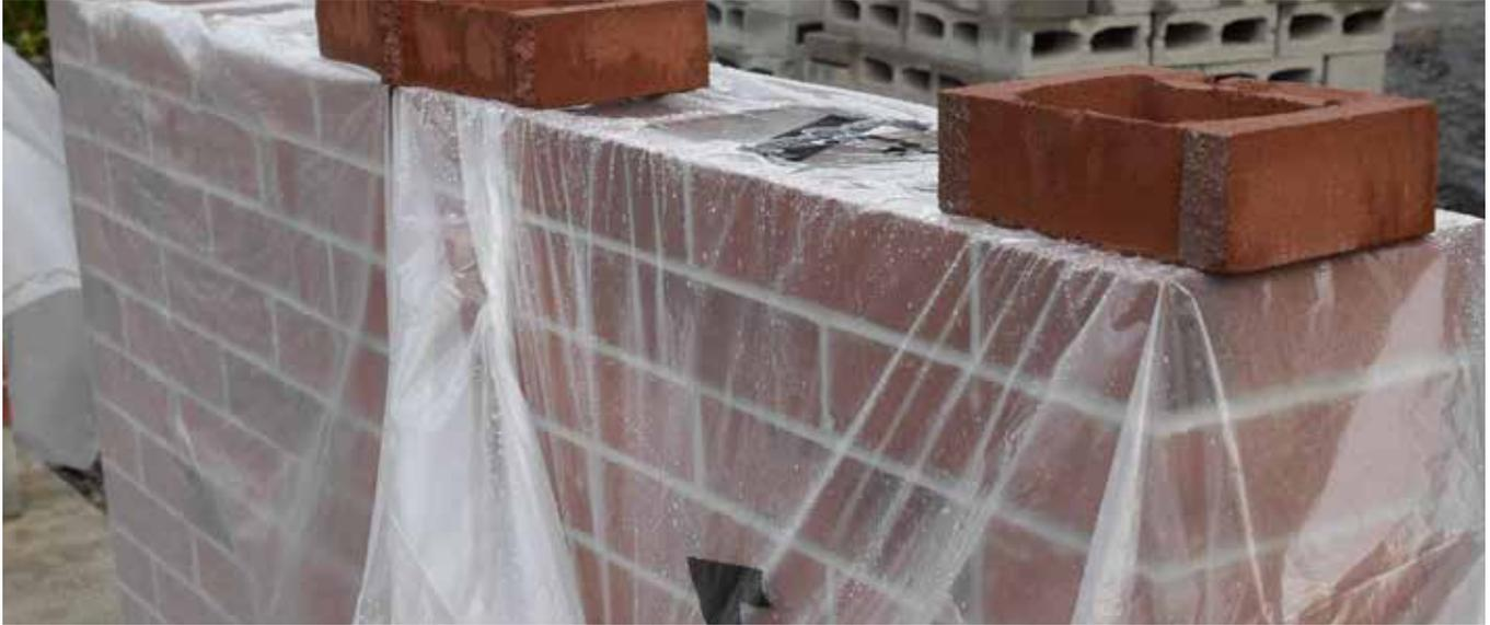
**T**o assure best results when building with architectural masonry, taking a few simple steps at the jobsite to protect the masonry materials and walls under construction will help deliver great results while reducing overall construction expense.
