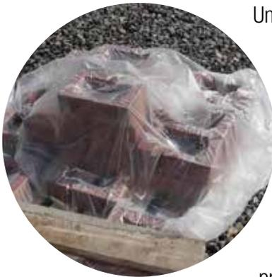
Units should be stored on pallets, and not directly on the ground. They should be adequately covered to prevent water absorption or staining from mud or other materials on the site.
