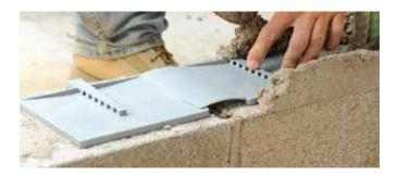
The mortar bed is placed along the course with the flashing units just as it would be normally. Care should be taken to clean out the weep spouts of the flashing units after the mortar joint is in place and is being tooled so that no mortar blocks the spouts. Mesh pieces are stuffed in the cores of the units above the flashing system to prevent mortar or grout droppings from plugging the system.
