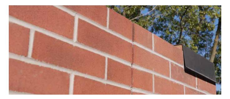
The sample panel will be used for final acceptance of the masonry work and must remain unharmed until the masonry is complete and accepted. The Masonry Code charging language states:
