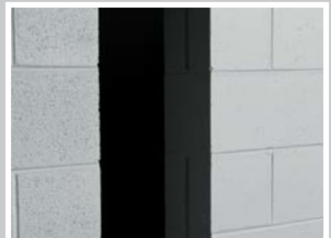
Ordinary CMU (left) and Spec-Surface, each with two coatings of paint.
